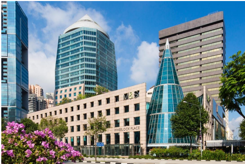
Photo: Wheelock Place
